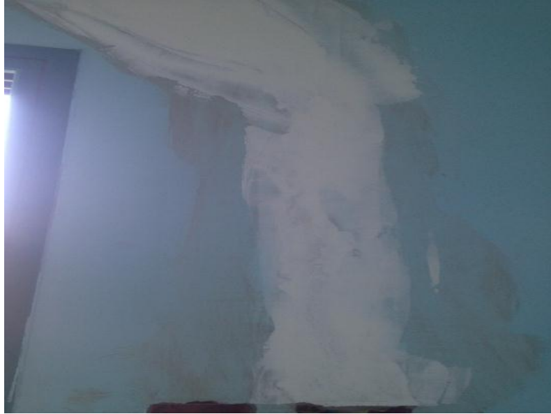
Figure 4.15 Preparing walls for maintenance
