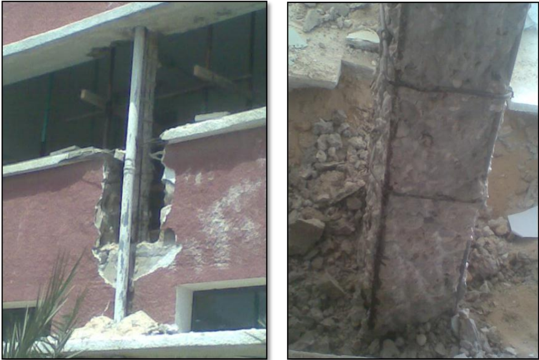
Figure 4.21 Preparing for jacketing
