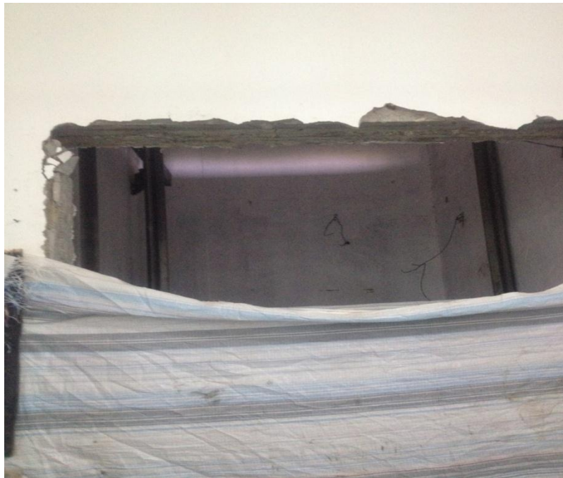
Figure 4.16 Installing new elevator
